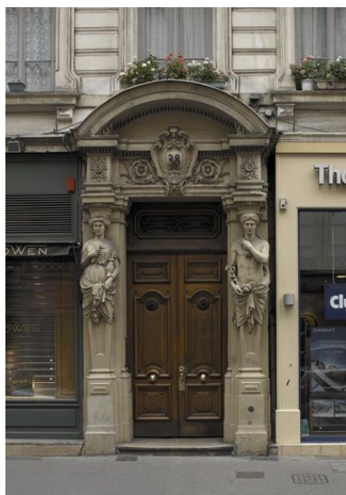
Façade principale, porte Phot. Didier Gourbin IVR82_20056901525NUCA
