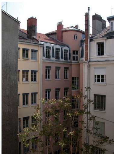
Elévations postérieures Phot. Maryannick Chalabi IVR82_20046904666NUCA
