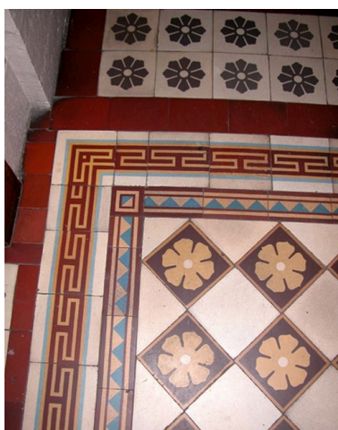
Pavement du vestibule Phot. Maryannick Chalabi IVR82_20046904512NUCA
