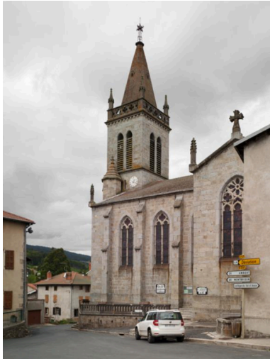
Vue partielle Phot. Christian Parisey IVR83_20156300291NUC4A
