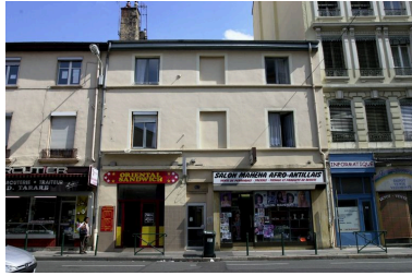
Elévation principale Phot. Maryannick Chalabi IVR82_20046904620NUCA
