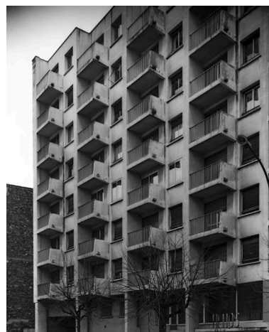
Façade du 46 boulevard Cote-Blatin Phot. Roger Choplain, Phot. Roland Maston IVR83_20006300413V
