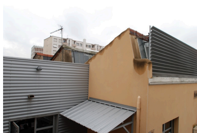
Toit shed Phot. Nadine Halitim-Dubois IVR82_20096901568NUCA
