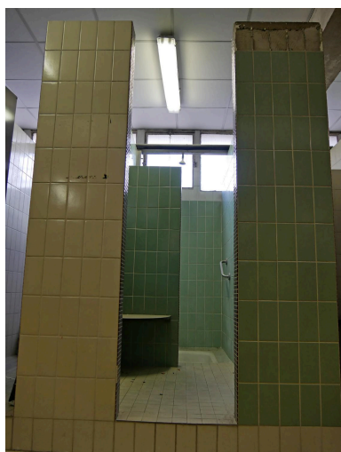
Cabine douche Phot. Nadine Halitim-Dubois IVR84_20256902099NUCA
