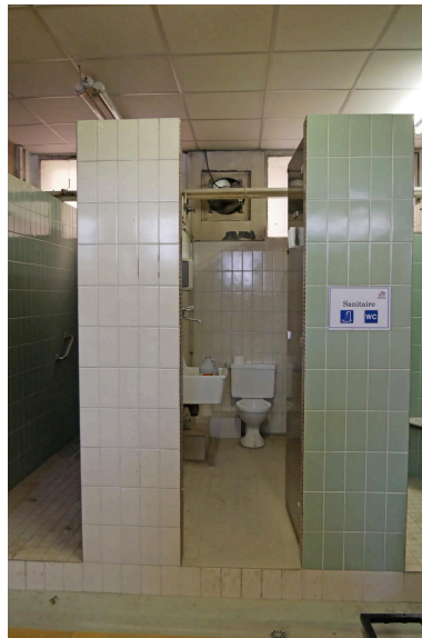
Cabine WC Phot. Nadine Halitim-Dubois IVR84_20256902094NUCA
