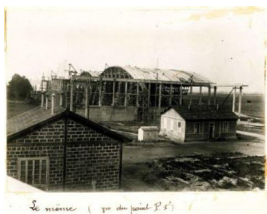
Hangar VI photo chantier ETs. Boussiron 1925 (ADR : 4535W47) Phot. Nadine Halitim-Dubois IVR84_20256900101NUC
