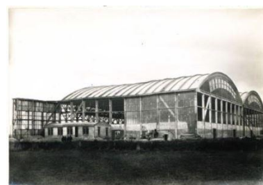
Hangar VI photo chantier ETs. Boussiron 1925 (ADR : 4535W47) Phot. Nadine Halitim-Dubois IVR84_20256900106NUC
