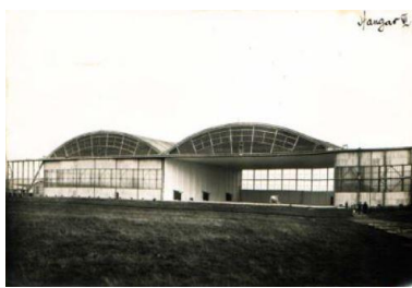
Hangar VI photo chantier ETs. Boussiron 1925 (ADR : 4535W47) Phot. Nadine Halitim-Dubois IVR84_20256900108NUC
