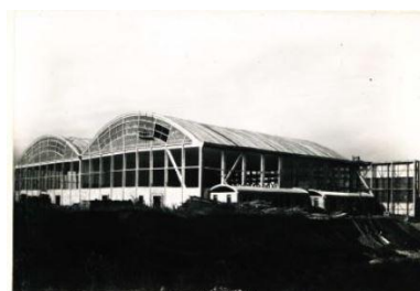
Hangar VI photo chantier ETs. Boussiron 1925 (ADR : 4535W47) Phot. Nadine Halitim-Dubois IVR84_20256900107NUC
