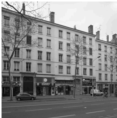
Elévation principale Phot. Eric Dessert IVR82_20056900634NUC
