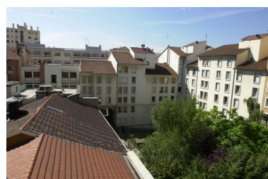
Elévations postérieures Phot. V. Baud IVR82_20046904997NUCA
