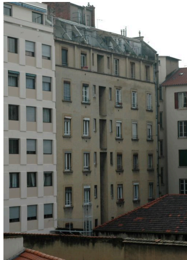
Elévation postérieure Phot. Maryannick Chalabi IVR82_20066903117NUCA
