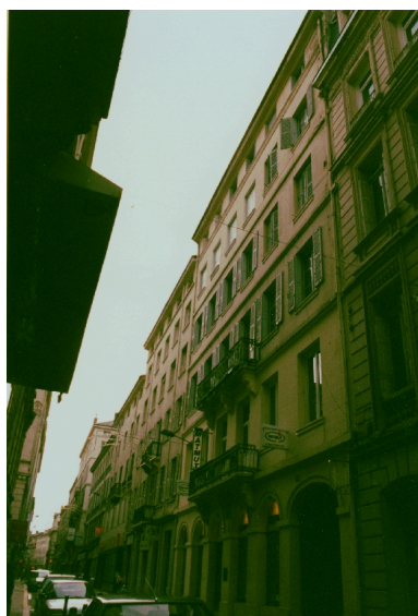
Façade principale Phot. Cendrine Sanquer IVR82_19974202017ZE
