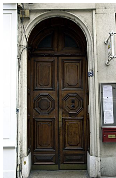
Façade principale, porte Phot. Maryannick Chalabi IVR82_20046900150NUCA
