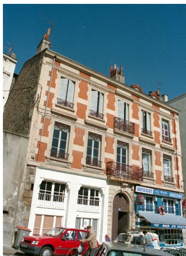
Façade principale Phot. Cendrine Sanquer IVR82_19974202096ZE
