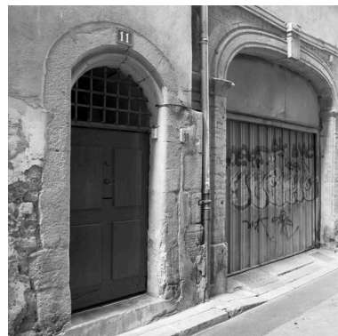
Façade, porte Phot. Didier Gourbin IVR82_20056901552NUC
