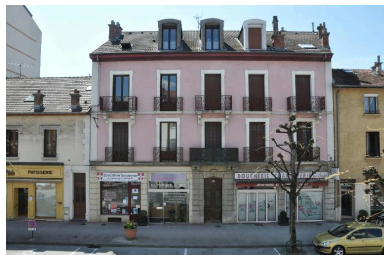
Façade principale Phot. Denys Harreau IVR82_20137300626NUCA
