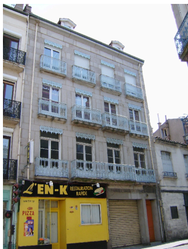
Elévation principale Phot. Cendrine Sanquer IVR82_20084200512NUCA
