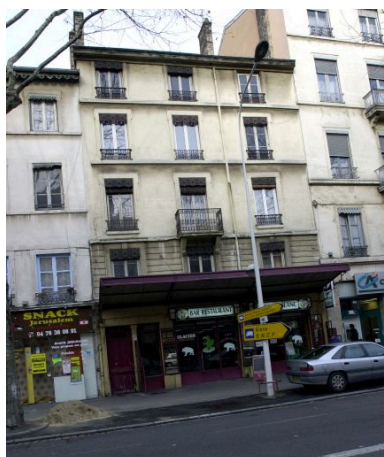
Elévation principale Phot. Maryannick Chalabi IVR82_20016900235NUCA
