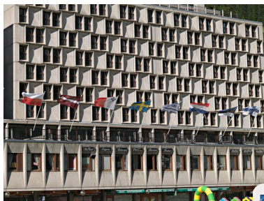
Façade principale Phot. Eric Dessert IVR82_20097400377NUCA
