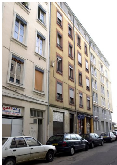
Elévation rue Denuzière Phot. Maryannick Chalabi IVR82_20016902122NUCA
