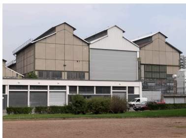
Grandes halles Phot. Eric Dessert IVR82_20096905641NUCA
