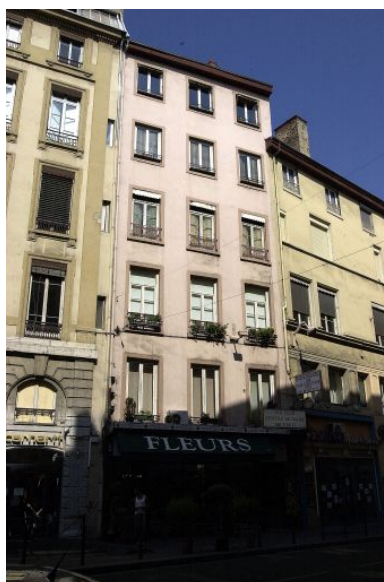
Façade principale Phot. Bernard Ducouret IVR82_20036901484NUCA
