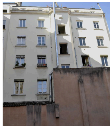
Elévation postérieure Phot. Magali Delavenne IVR82_20156901225NUCA
