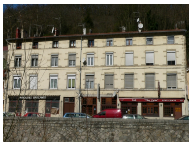
Façade principale Phot. Isabelle Dupuis IVR82_20093800329NUCA
