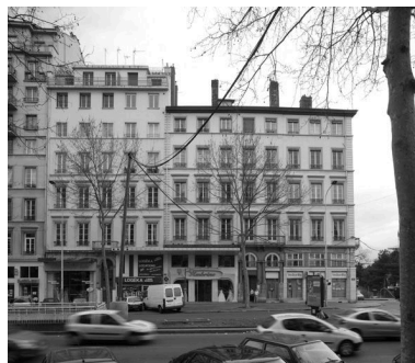
Elévation principale Phot. Eric Dessert IVR82_20056900657NUC
