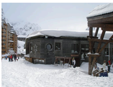
Elévation nord Phot. Jean-François Lyon- Caen, Phot. C. Salomon-Pelen IVR82_20087400503NUCA
