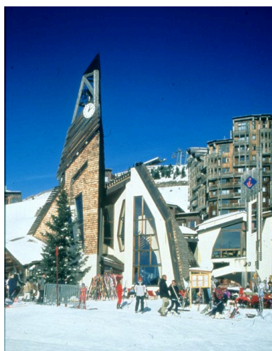
Façade sud Phot. Jean-François Lyon- Caen, Phot. C. Salomon-Pelen IVR82_20087400499NUCA
