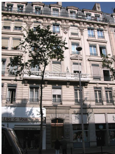
Elévation principale Phot. Maryannick Chalabi IVR82_20046904544NUCA
