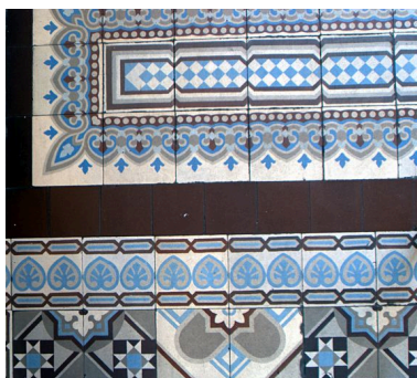
Carrelage en carreaux de ciment, vestibule Phot. Maryannick Chalabi IVR82_20116904043NUCA
