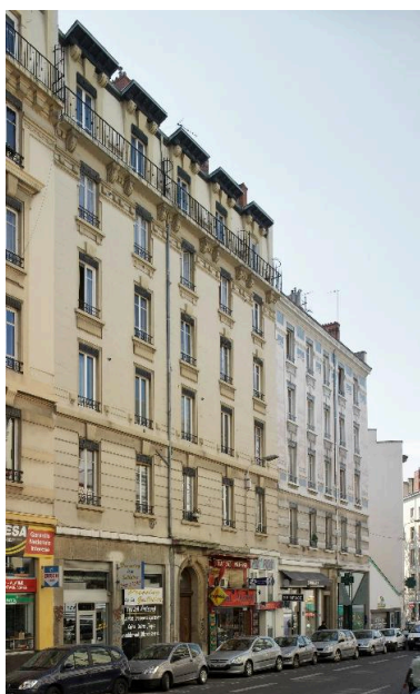
Elévation principale Phot. Eric Dessert IVR82_20076902429NUCA
