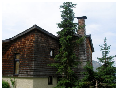
Elévation nord Phot. Jean-François Lyon- Caen, Phot. C. Salomon-Pelen IVR82_20087400168NUCA
