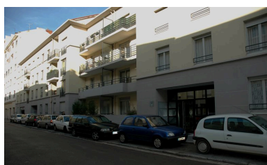
Elévation, rue Alphonse-Daudet Phot. Maryannick Chalabi IVR82_20076900384NUCA
