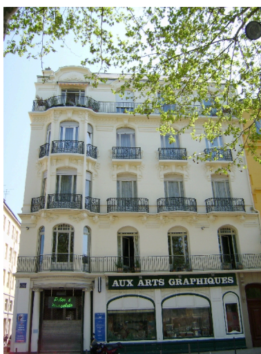
Façade, place Jean-Jaurès Phot. Cendrine Sanquer IVR82_20084200511NUCA
