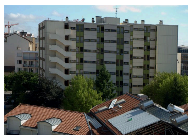
Elévation postérieure Phot. Maryannick Chalabi IVR82_20086900883NUCA
