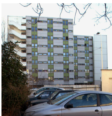
Elévation antérieure Phot. Maryannick Chalabi IVR82_20126902457NUCA
