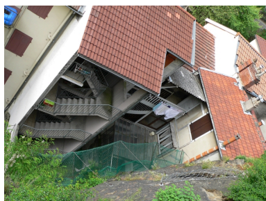
Distribution arrière Phot. Isabelle Dupuis IVR82_20093800519NUCA
