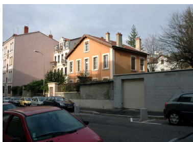
Bow-window et balcon, élévation sud Phot. Véronique Belle IVR82_20066900777NUCA
