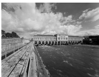
Façade aval Phot. Eric Dessert IVR82_20026904308V
