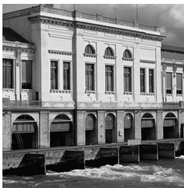
Corps central Phot. Eric Dessert IVR82_20026904317X
