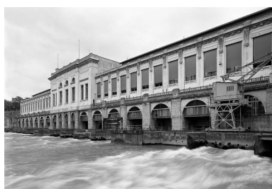
Façade aval Phot. Eric Dessert IVR82_20026904306P
