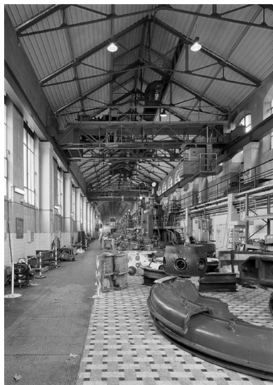
Salle des machines Phot. Eric Dessert IVR82_20026904349P
