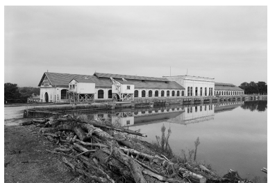
Façade amont Phot. Eric Dessert IVR82_20026904322P
