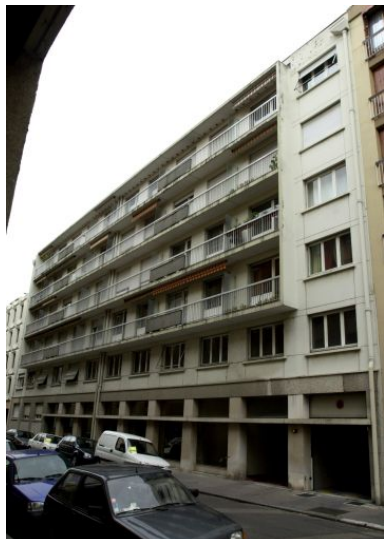
Elévation principale Phot. Maryannick Chalabi IVR82_20016902407NUCA
