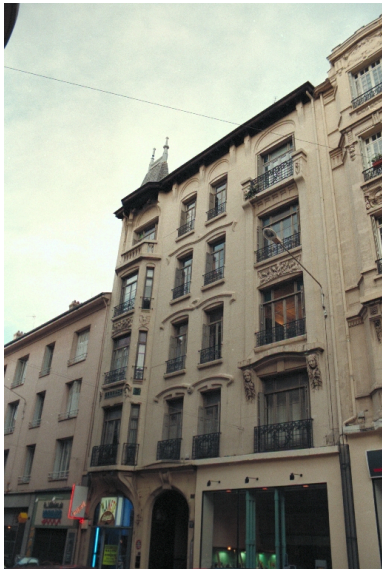
Façade principale Phot. Cendrine Sanquer IVR82_19974202097ZE
