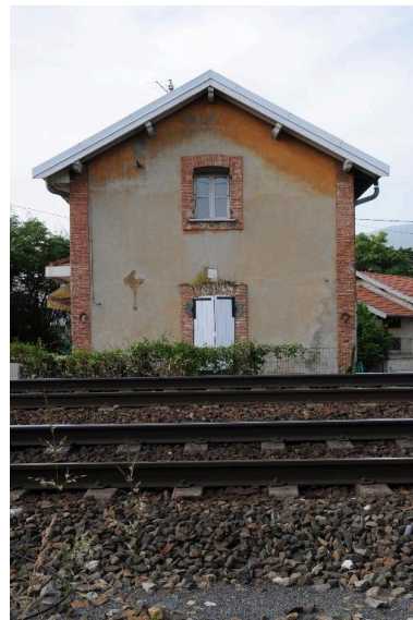
Pignon nord Phot. Denys Harreau IVR82_20147300858NUCA
