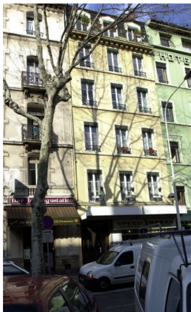
Elévation principale Phot. Maryannick Chalabi IVR82_20016900248NUCA
