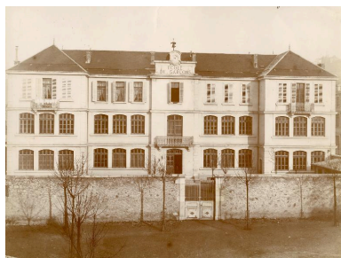
Façade principale, 1889 Repro. Denys Harreau IVR82_20157301075NUCB
