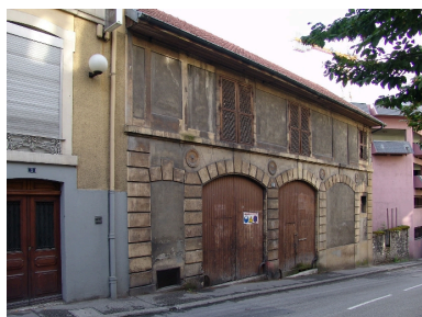
Façade Phot. François Fouger IVR82_20057300634NUCA
