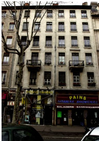
Elévation principale Phot. Maryannick Chalabi IVR82_20016900260NUCA
