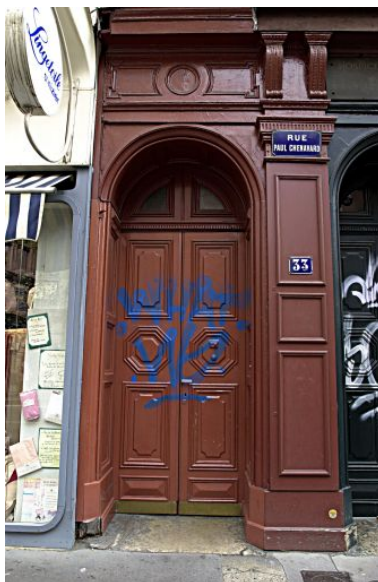
Façade principale, porte Phot. Maryannick Chalabi IVR82_20046900161NUCA
