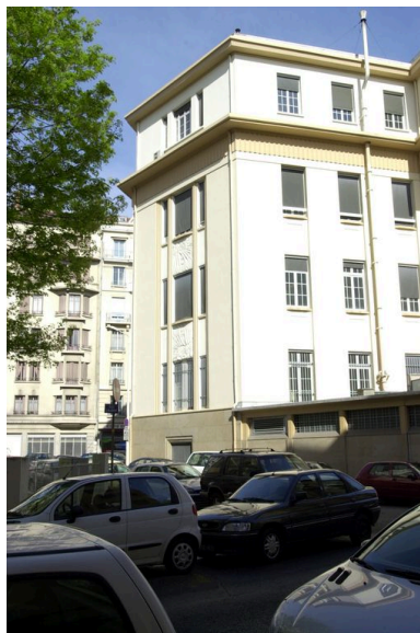
Elévation sud Phot. David Chevallier IVR82_20046902090NUCA
