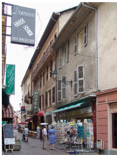
Façade Phot. François Fouger IVR82_20057300523NUCA
