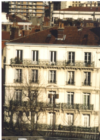
Façade principale Phot. Cendrine Sanquer IVR82_19974202054ZE
