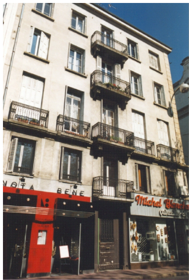
Façade principale Phot. Cendrine Sanquer IVR82_19974202047ZE
