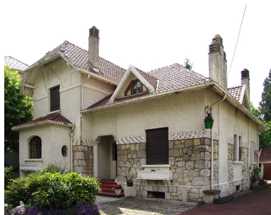
Façade principale Phot. François Fouger IVR82_20097300604NUCA
