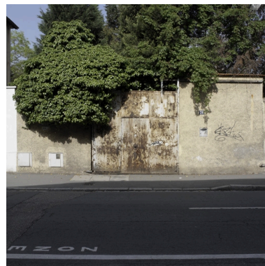
Entrée marchandise Phot. Eric Dessert IVR82_20056900110NUCA
