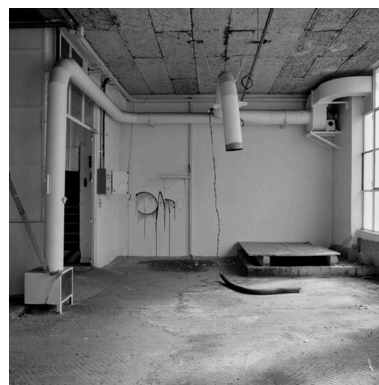
Structure de ventilation Phot. Eric Dessert IVR82_20066902844X
