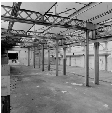
Extension de 1960 Phot. Eric Dessert IVR82_20066902850X
