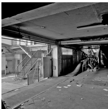
Extension de 1960 Phot. Eric Dessert IVR82_20066902852X
