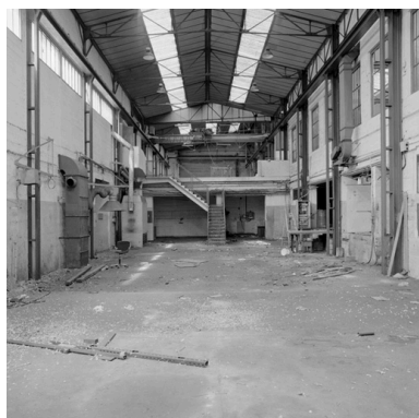
Extension de 1960 Phot. Eric Dessert IVR82_20066902849X
